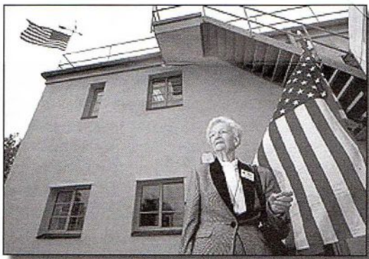
Charlotte Shower officially opens the extensively restored control tower at Rackheath, which will now be used as an office suite.
